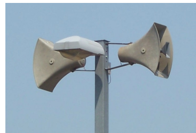
Figure 25.15: These speakers are shaped to take advantage of diffraction for sound waves. The narrower the opening, the wider the diffraction pattern. The speakers are designed to diffract sound waves horizontally, where they can be heard by people on a train platform. Photo credit: A. Duffy.
